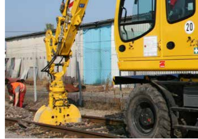
Safe track construction – for man and machine.
